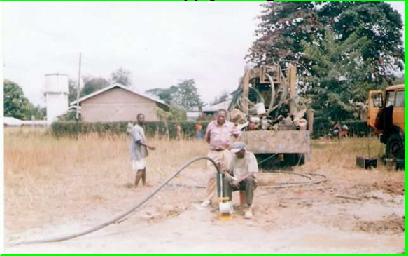
Drilling a 60m bore-hole at Lugala
