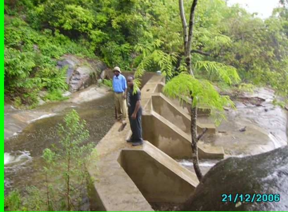
Completed intake structure for Chita Village
