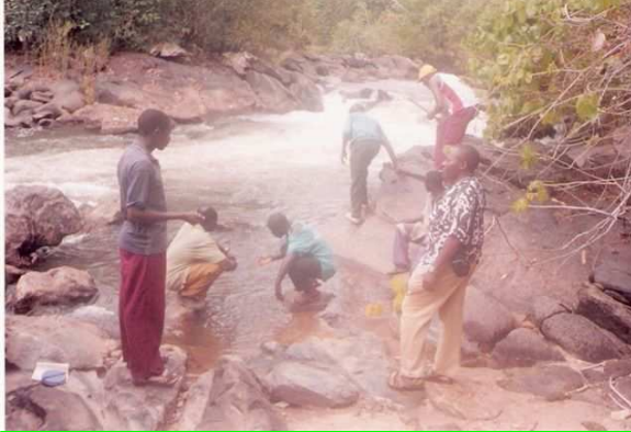
Identification of intake point for Matema Village
