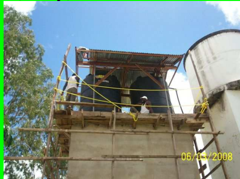
Construction of 10,000 liters tank at Lugala
